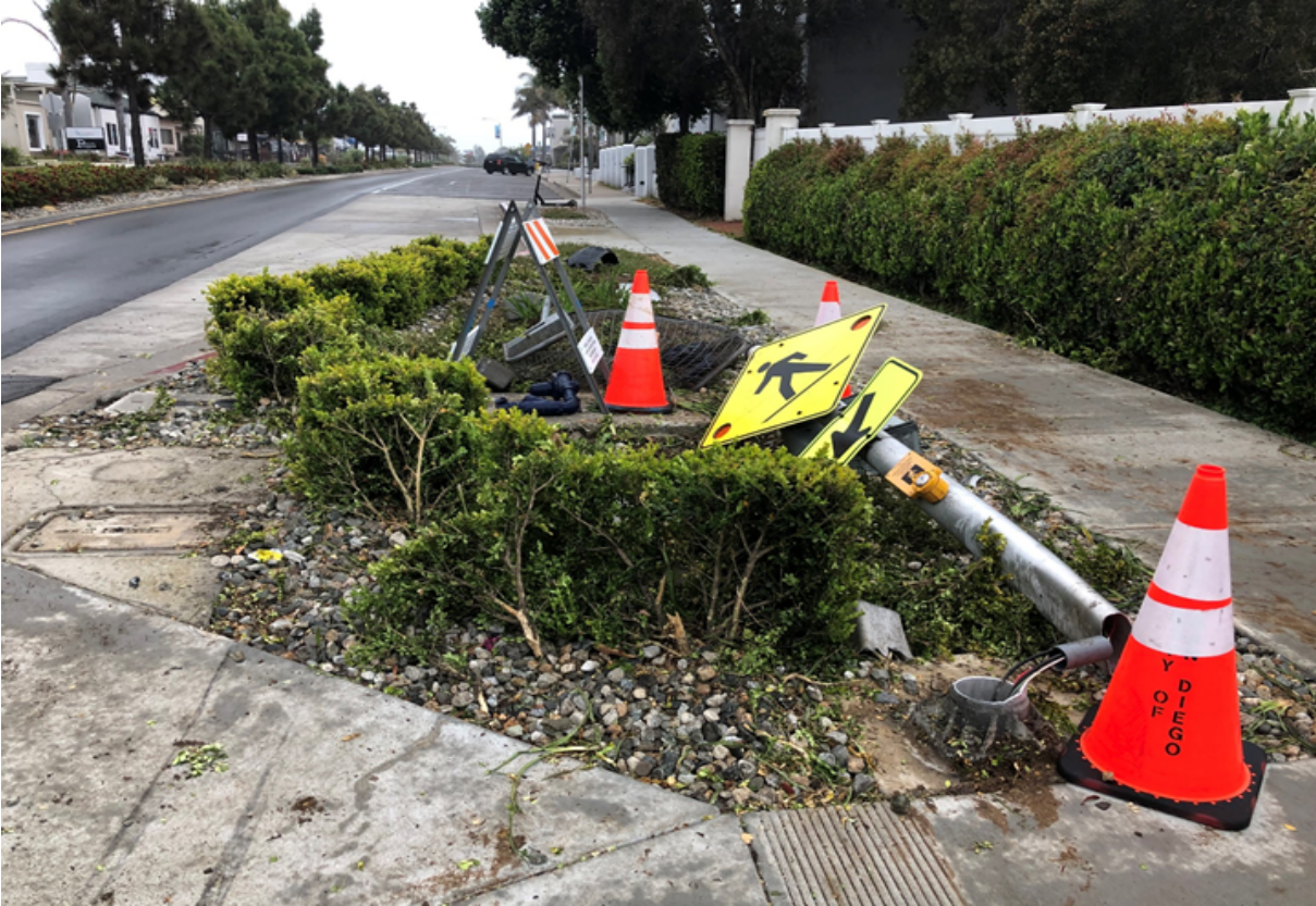
Part of the damage from an accident at the south west corner of La Jolla Blvd. and Camino de la Costa including a sheered off pedestrian crossing signal, City water backflow valve and protective cage, and irrigation controller.
